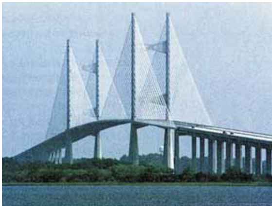
写真-9.3 Dames Point bridge 1)
