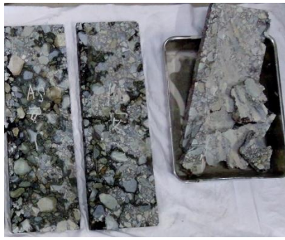
Photo.1 Damaged asphalt mixture
