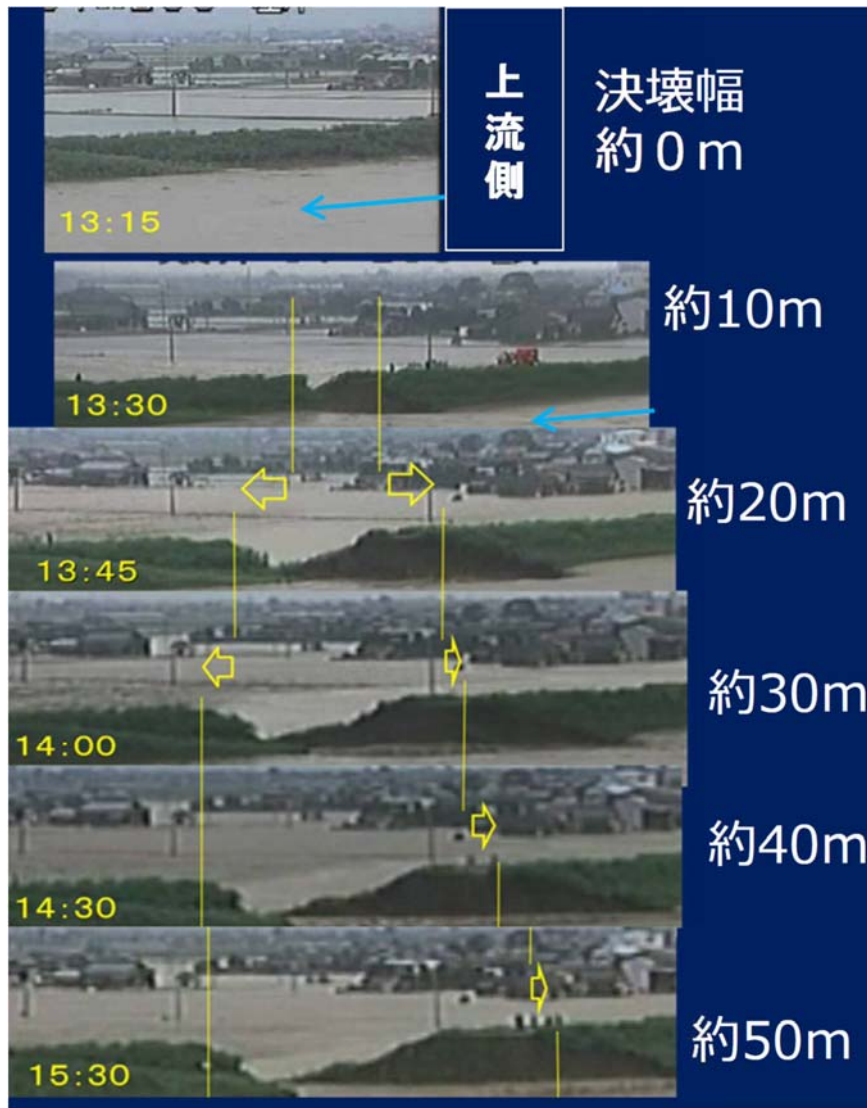
Figure 1-13 the failure process of the levee in Yabegawa River in Fukuoka, 2012 [12]
