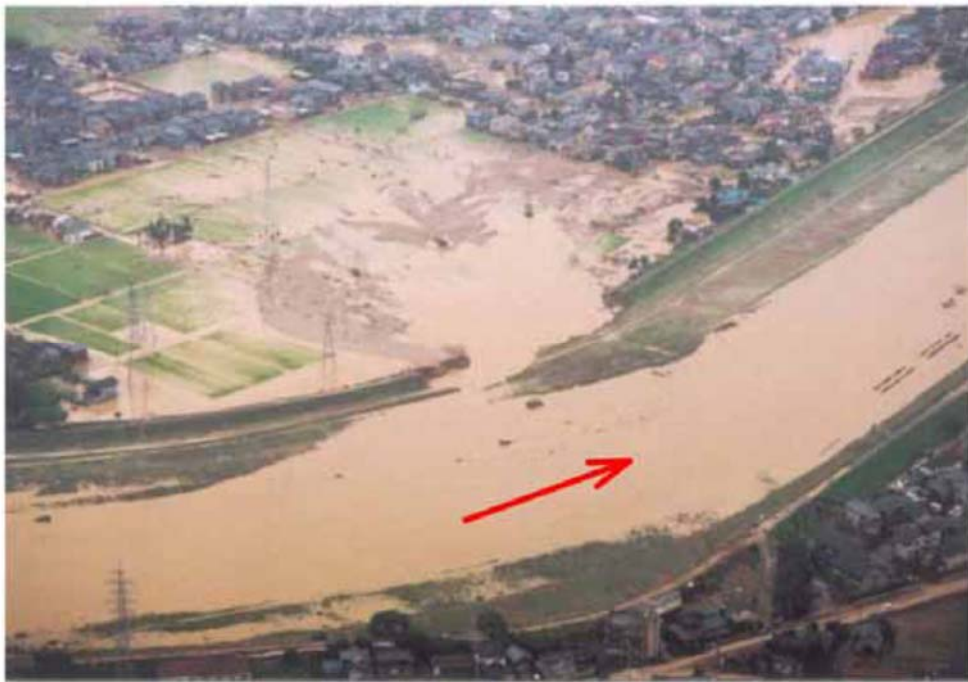
Figure 1-11 the failure situation in Shinanogawa River in Nigata, 2004 [7]
