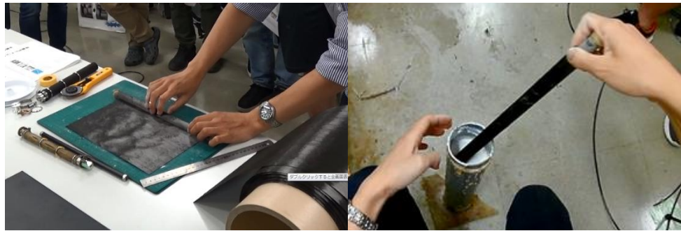
(c) Wrap the reinforcing fiber
