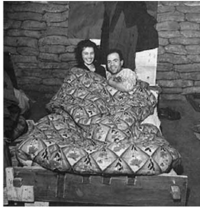
Figure 4-2: 'West End Shop Basement Shelter', November 7, 1940.
